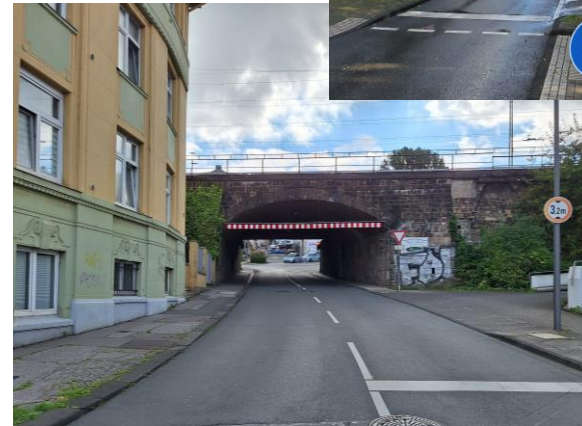
Railway Bridge, Wuppertal, Germany
